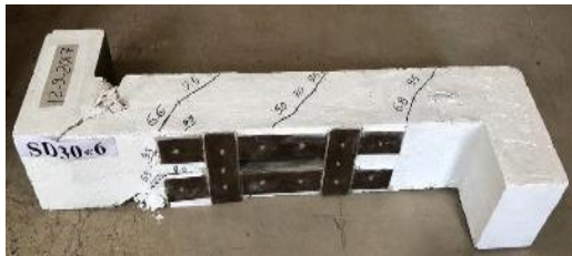
(a) Crack pattern for SD30x6
