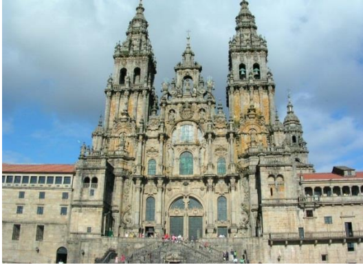
Figure 7- The Obradoiro façade (north façade) [17]
