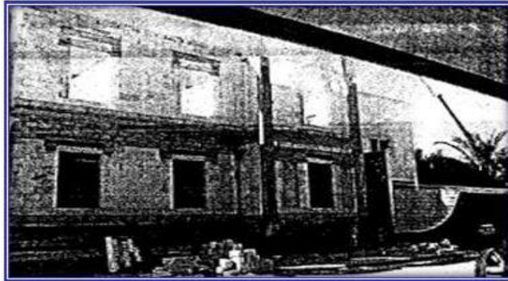
Figure 1 General view of the building
